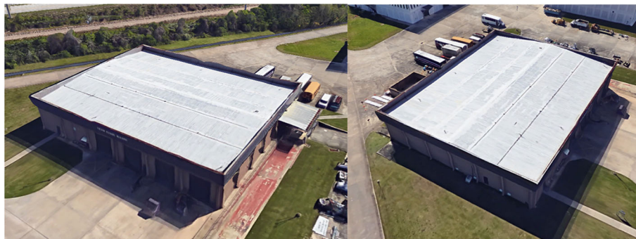
Fig. 5 A low-rise building with gable roof and perimeter parapet, Baton Rouge, Louisiana (Dimensions: 163 ft. \times 130 ft. \times 21.5 ft.)
